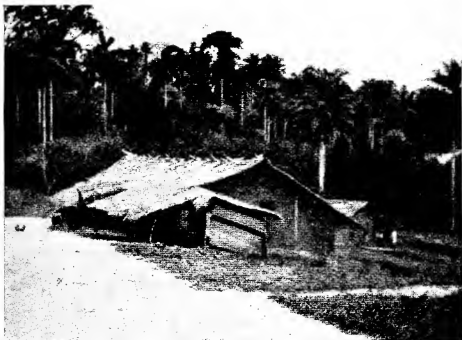
COURT HOUSE AT IKOTOBONG
